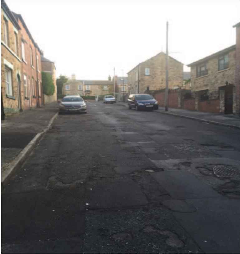
Figure 4 View further up Parsonage Street
