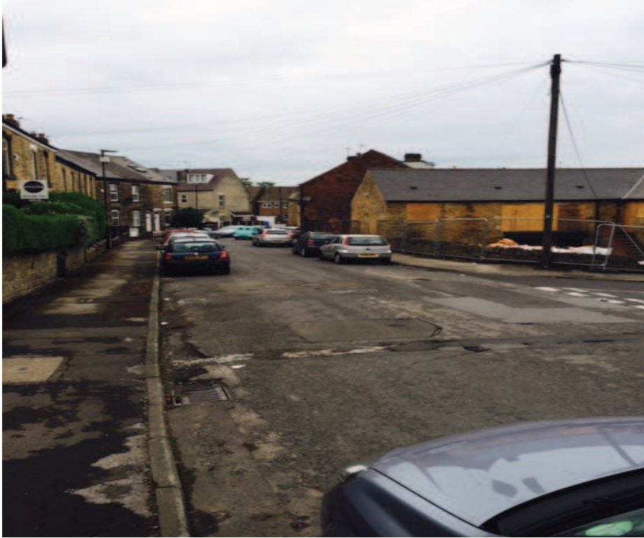
Figure 3 View eastwards along frontage of site on Parsonage Crescent
